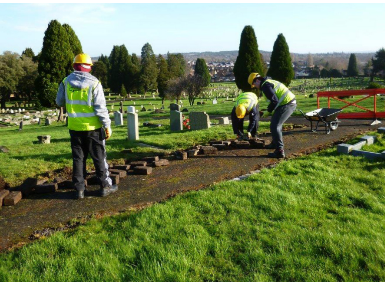
Skilled Up programme repairing pathways
