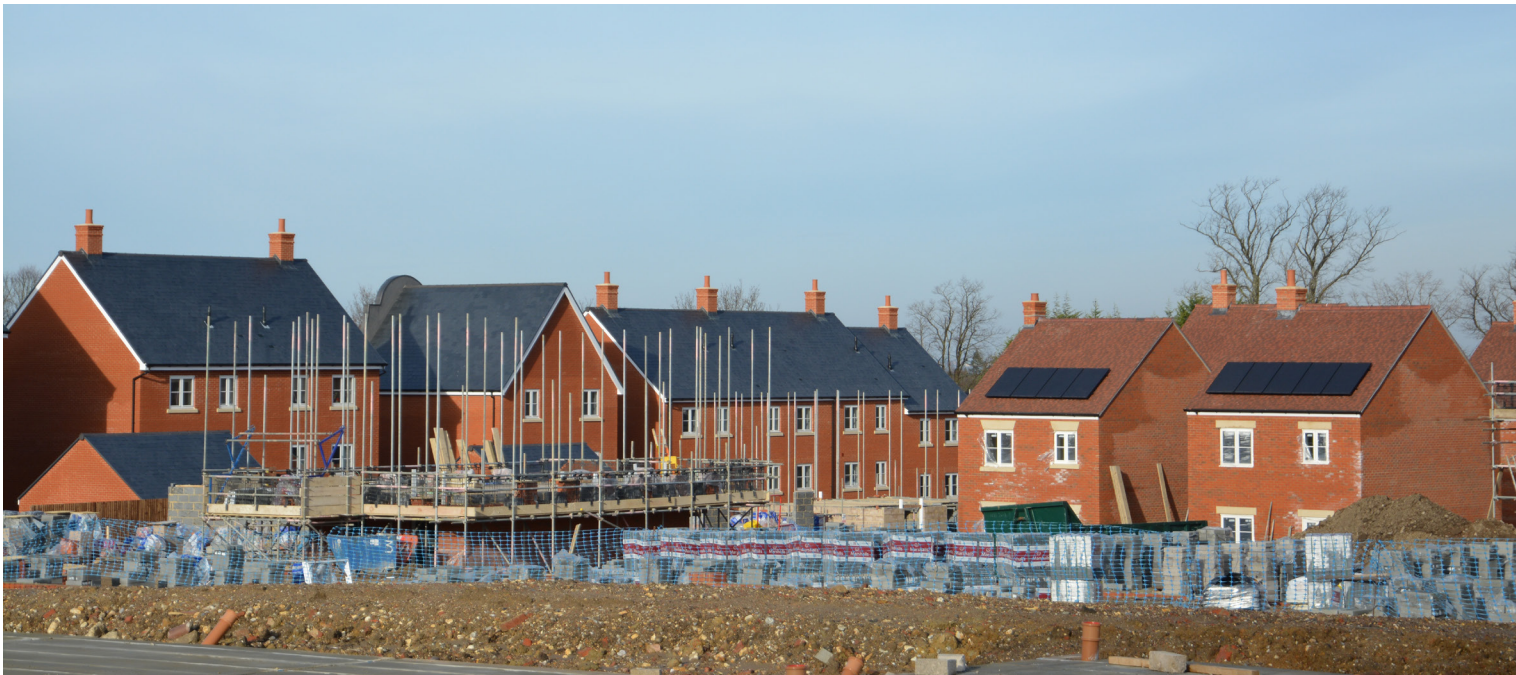
Wellesley's Maida development under construction
